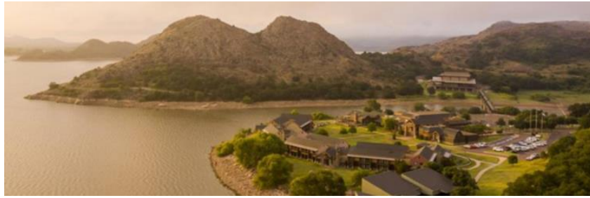
Figure 22: Overhead view of the Quartz Mountain State Park Lodge and surrounding landscape in Lone Wolf, Oklahoma.
